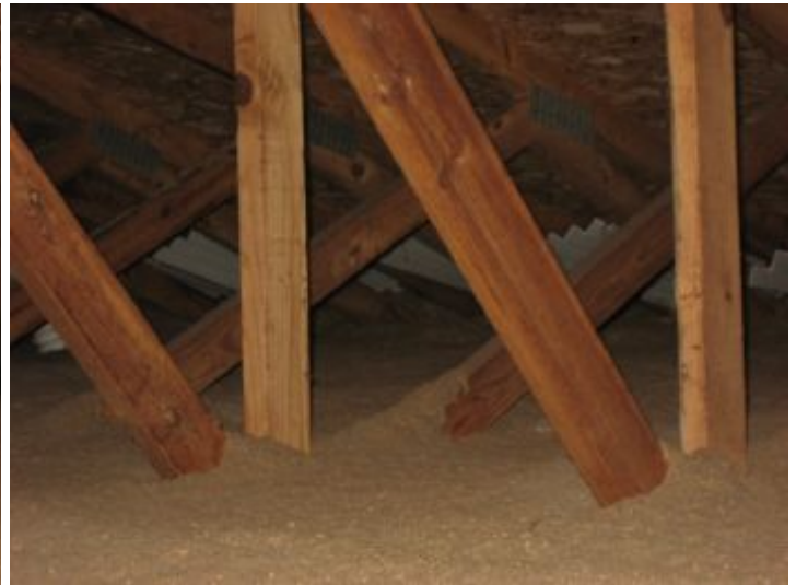
Insulation coverage in attic
