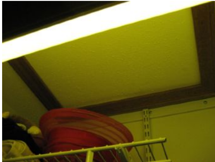
Scuttle Hole Access to Attic
